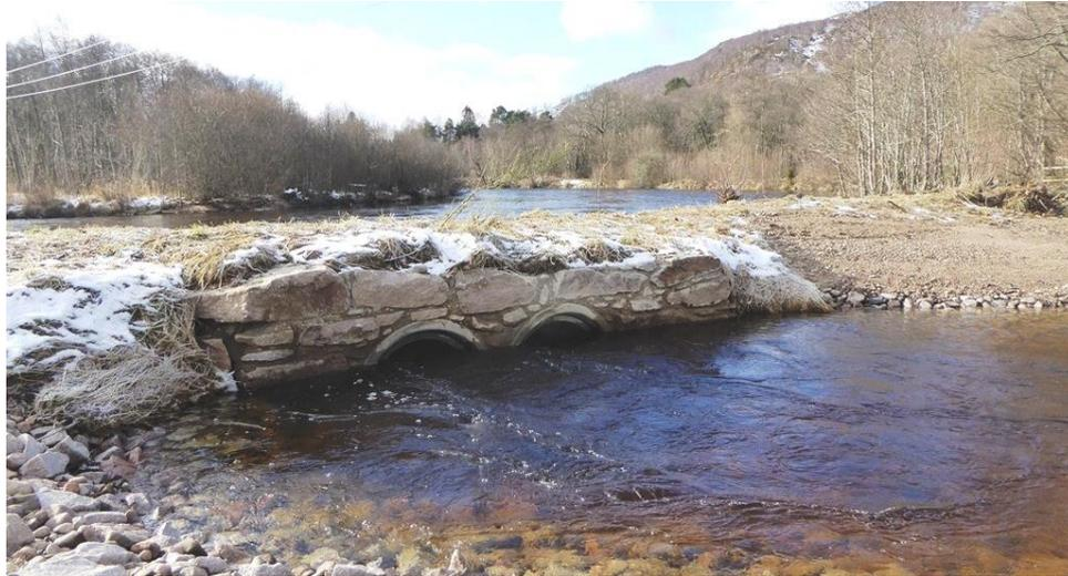
The channel was blocked off with rock armour around 50 years ago to reduce flood and erosion risk to nearby properties. Until the restoration works took place in Feb 17, flow only entered the channel during spate conditions when the main stem of the Spey overtopped the bank and the whole area flooded. Out with these events, the watercourse was stagnant or had minimal flow, leading to poor habitat which was a dank, often smelly ditch rather than a gently flowing burn.
